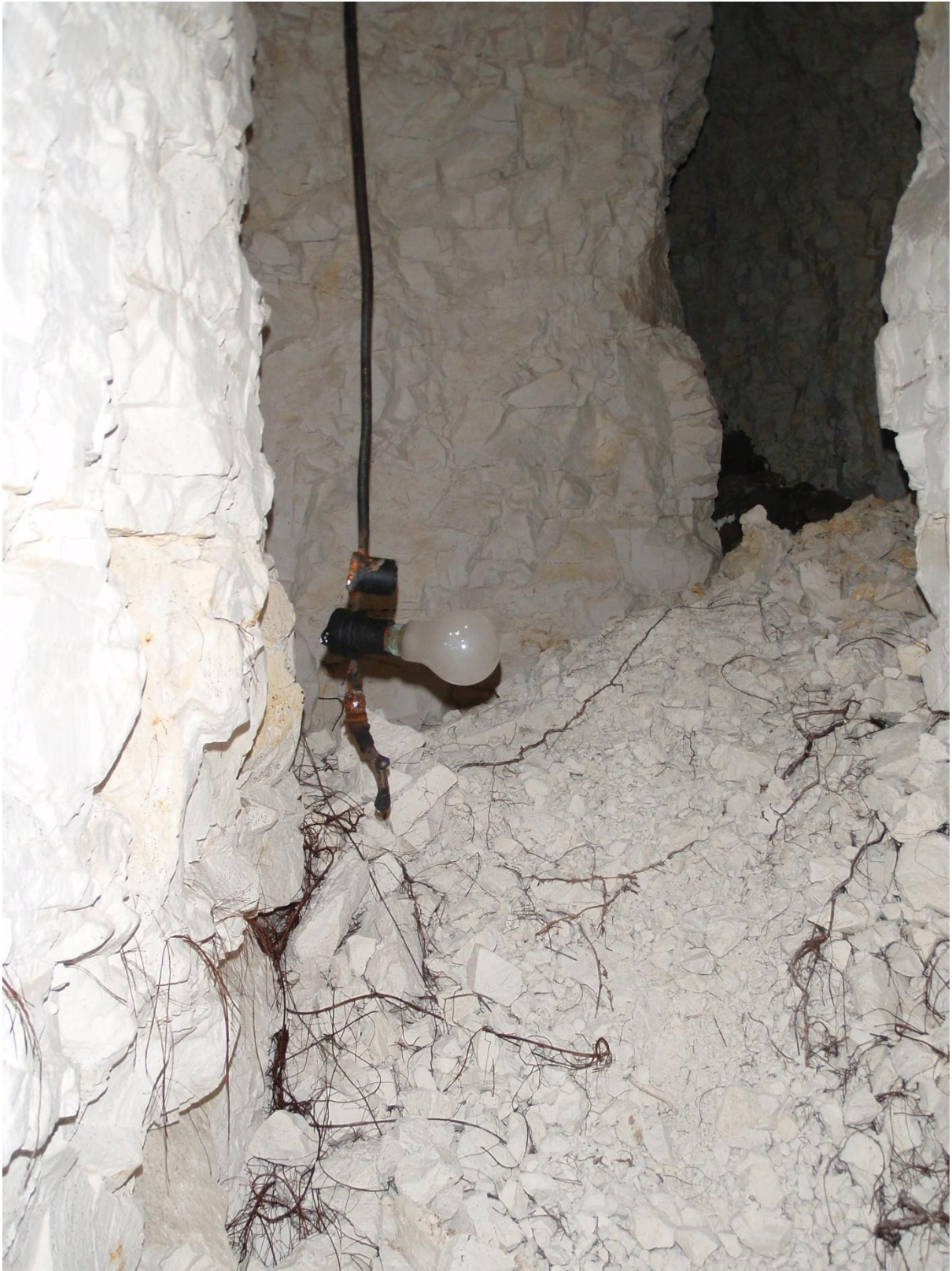
Plate 2. Bomb baffle on the west staircase,(with collapsed ceiling).
